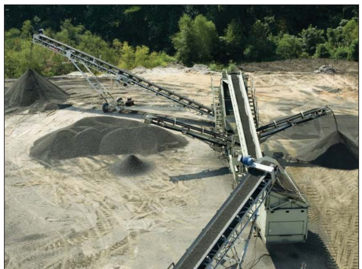
Then it moves up to a PEP Vari-Vibe® double-deck screen where it is separated—or fractionated—into three different sizes. The aerial view (below) provides a view of the three stockpiles that are the result of the Fold 'n Go screening plant's efficient process.
